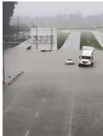
Figure 12: Floodwaters on US-378 in Sumter County
