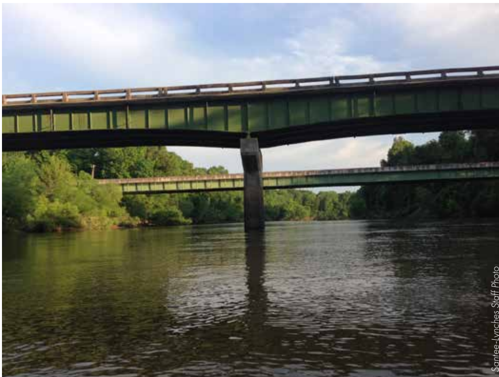
Figure 91: US-378/76 Bridge over the Wateree River
