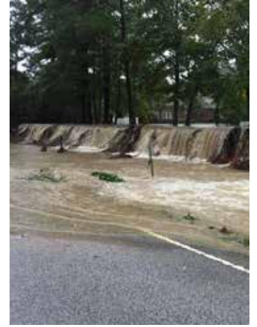
Figure 13: Floodwaters wash out a roadway in Sumter County
