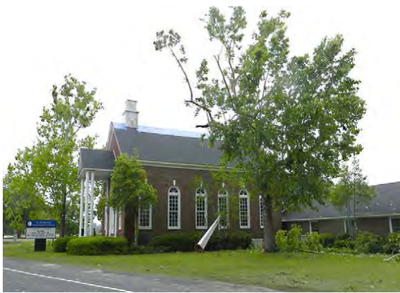
Figure 6 - Clarendon County Severe Thunderstorm (church steeple off with downed trees)
