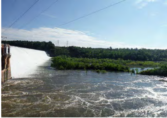
Figure 5 - Dam Failure – Water overtopping the Lake Wateree Dam
